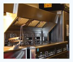
ing oil caught fire and flames were sucked up into the hood, thus spreading quickly. This risk is significantly reduced when fat particles are removed from the air, says lb Pedersen.
